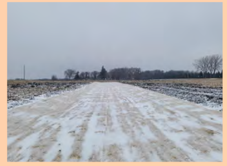
Completed grassed waterway with erosion control blanket.
