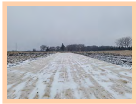
Completed grassed waterway with erosion control blanket.
