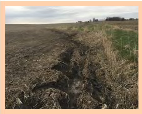
Erosion along an old grassed waterway before it was reconstructed.
