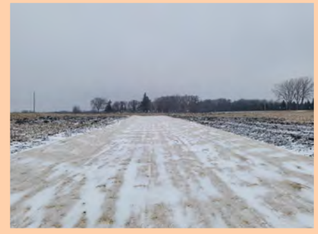
Completed grassed waterway with erosion control blanket.
