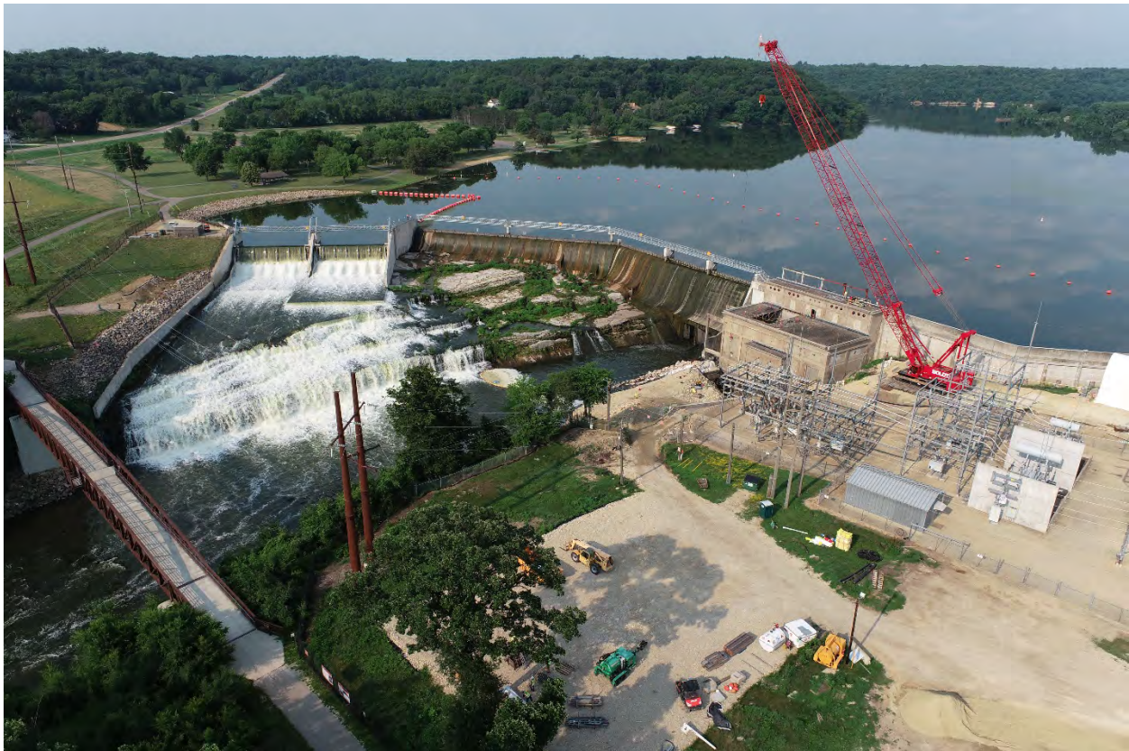
Figure 4-2: Lake Byllesby Dam
