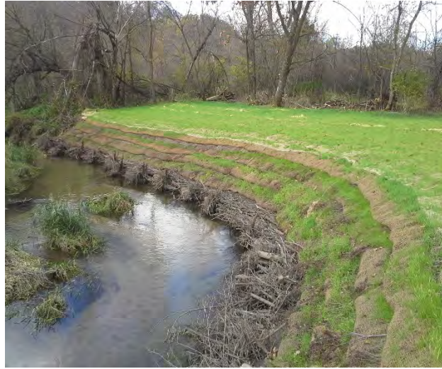
Figure 2-25: Streambank Restoration – Pine Creek
