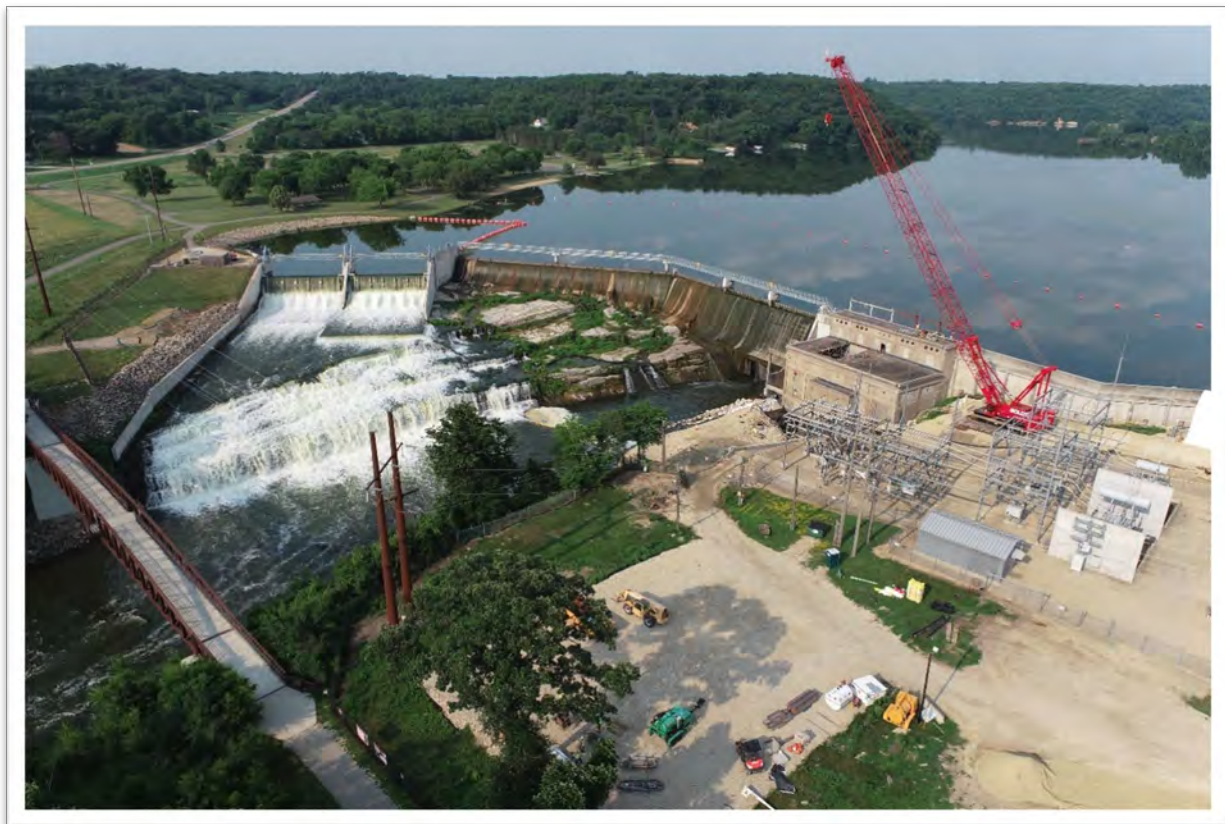
Figure 2-8: Lake Byllesby Dam
