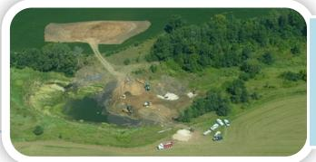
Construction of a grade stabilization structure in Goodhue County that will slow the flow of water and reduce sediment downstream.
