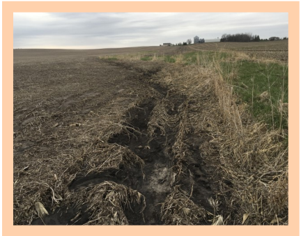
Erosion along an old grassed waterway before it was reconstructed.
