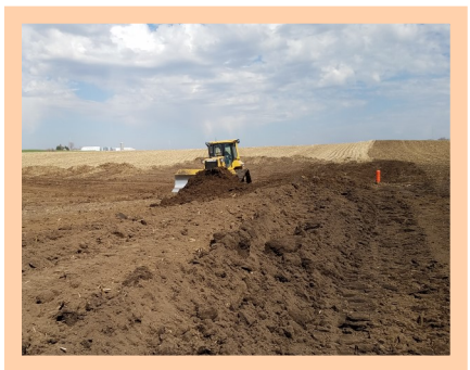
Moving dirt for a Water and Sediment Control Basin at Rodney Weber project
