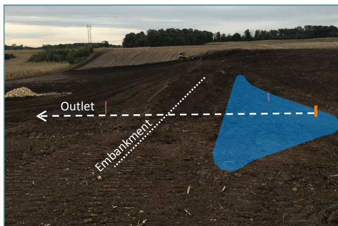
Embankments were constructed for each basin to store the runoff while it is slowly released through the outlet and underground tiles.
