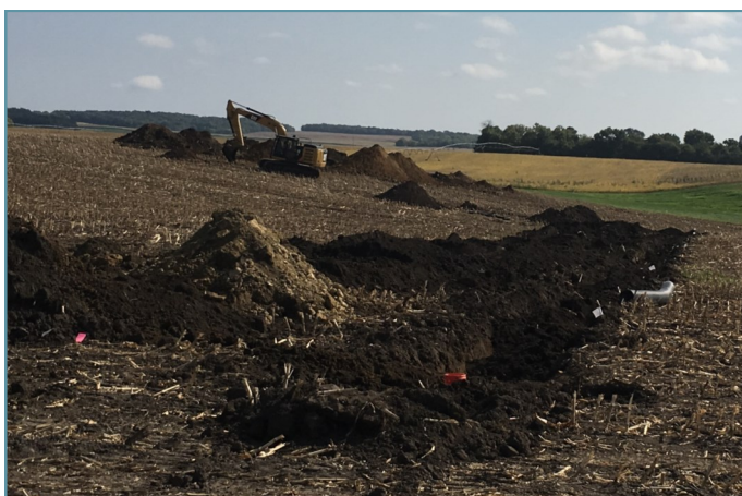
Underground tiles with surface inlets were installed to slowly discharge surface water runoff to a stable outlet.
