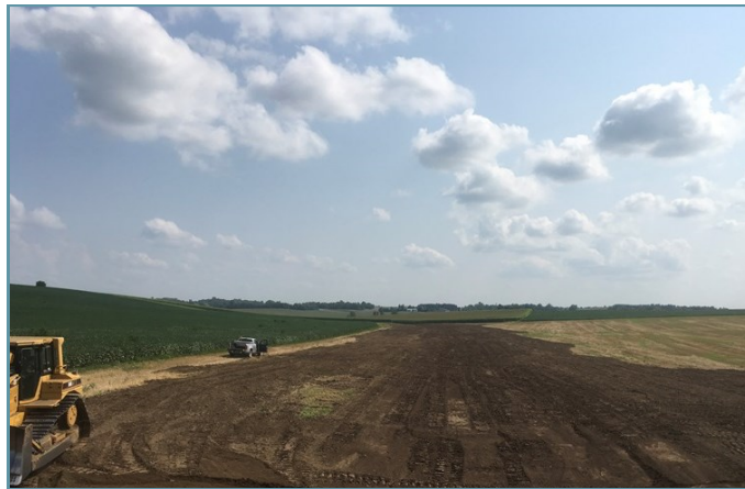
Accumulated sediment was excavated and the waterway was graded.
