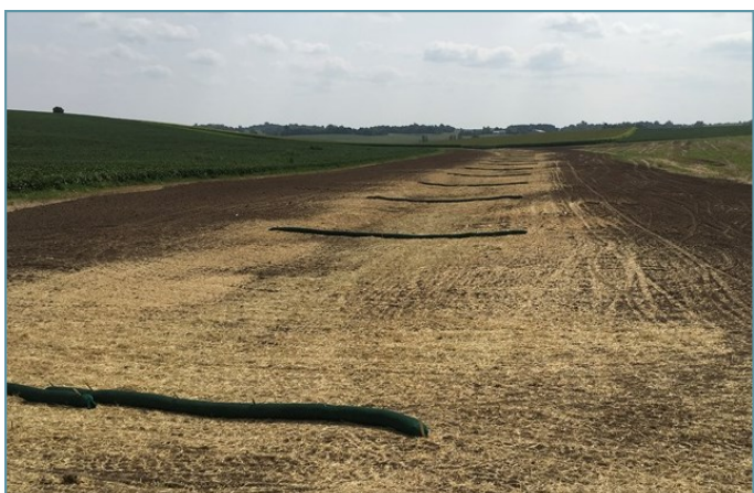
Temporary bio-logs were installed to slow down and disperse runoff from large rain events.
