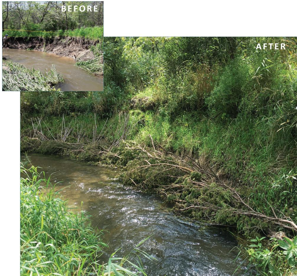
**PROJECT:** Five eroding streambanks along Trout Brook in Miesville Ravine Park Preserve were stabilized. The project used cedar tree revetment, live stakes, and sod mats to stabilize the eroding streambanks. The projects were completed by crews from the Conservation Corps of Minnesota and Iowa.
