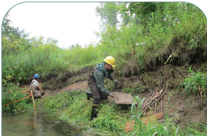
Harvested sod mats were anchored on the face of the bank to provide rapid establishment of vegetation.
