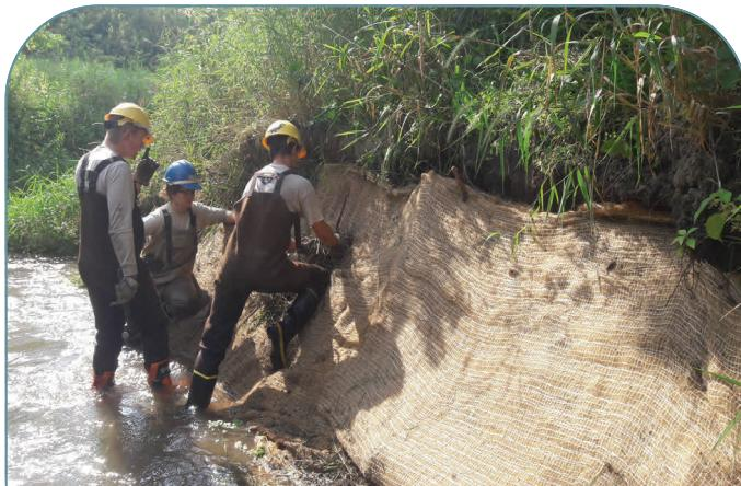
Natural erosion control netting was installed on exposed portions of the bank to prevent further face erosion.
